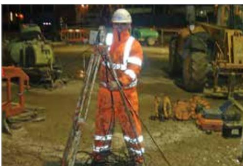
**JFTS provided sonic logging on a range of deep piled foundations and diaphragm walls at four different underground stations as part of the prestigious Crossrail transport scheme in London.**
